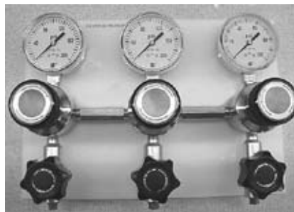
three-regulator panel - inlet may be from the left or right
